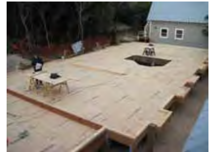
1st Floor installation
