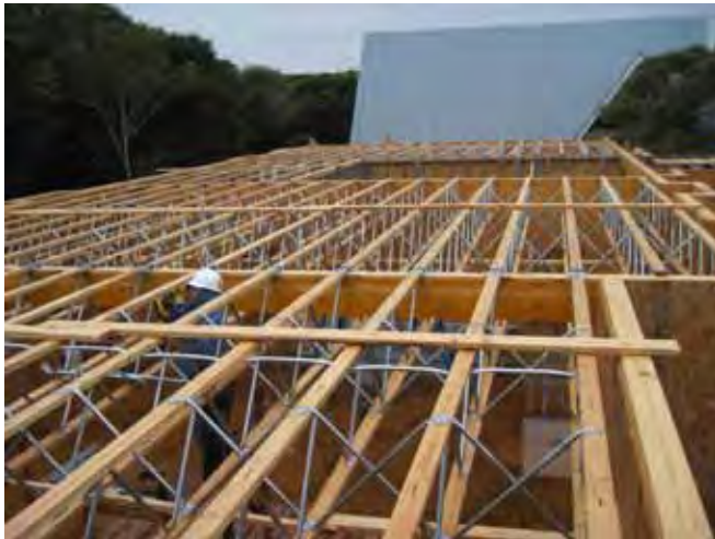
2nd Floor Trusses
